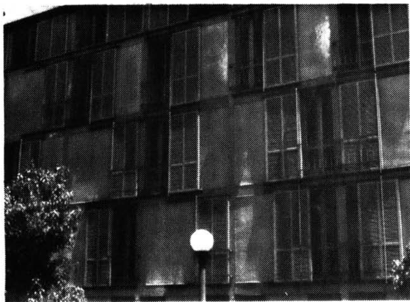
shutters on a building at Stanford University, CA.
