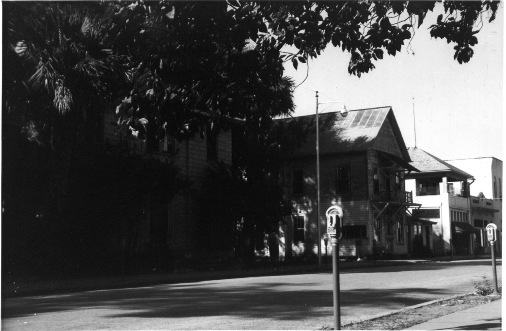
9. BUILDINGS OPPOSITE THE SITE LOOKING NORTHWEST
