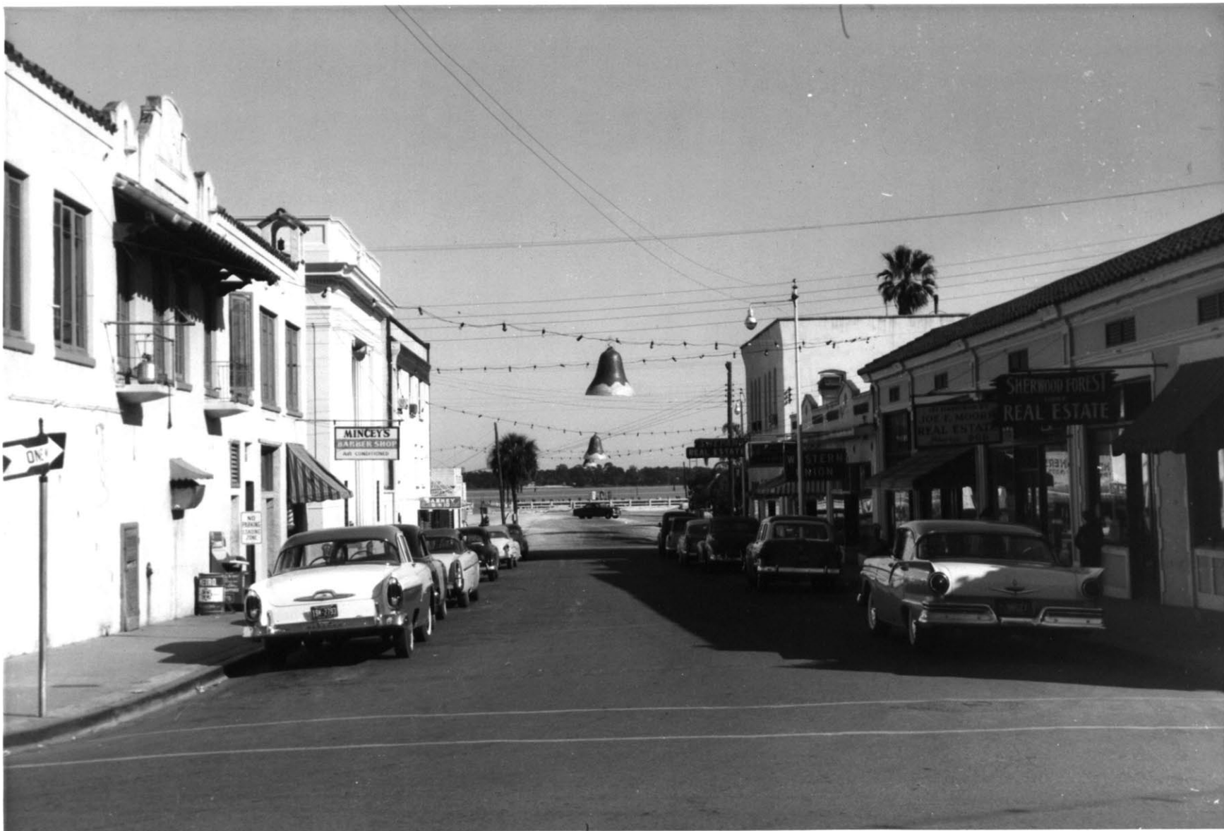
S. HARRISON AVENUE LOOKING EAST
