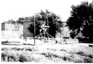
The Tower takes shape 72
