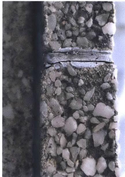
DETAIL OF MO-SAI PANEL AGGREGATE AND JOINT CONDITION
