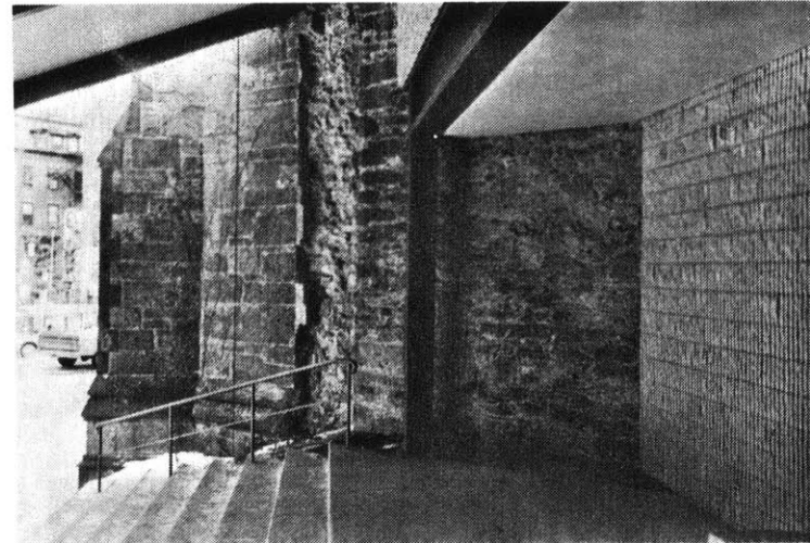
First and Second Church, Entry at tower
