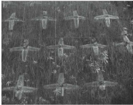
01_GROUND ANCHORS / CONCRETE
