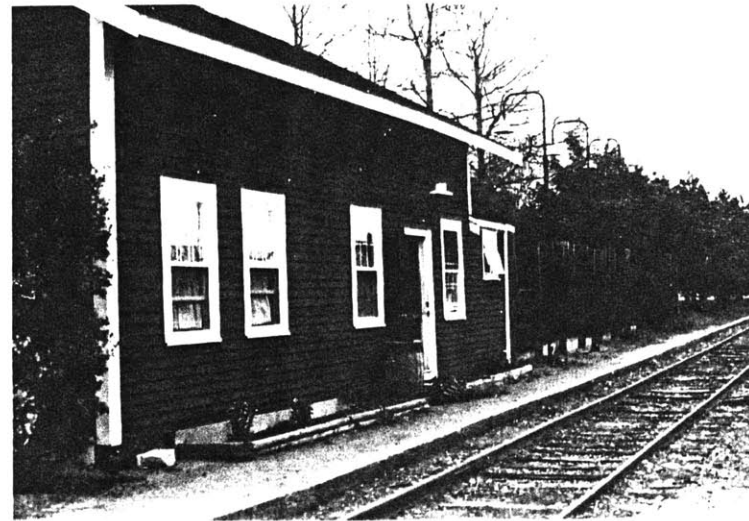
Figure 6-4: Railroad tracks and Upper Falls depot (5/4/95).
