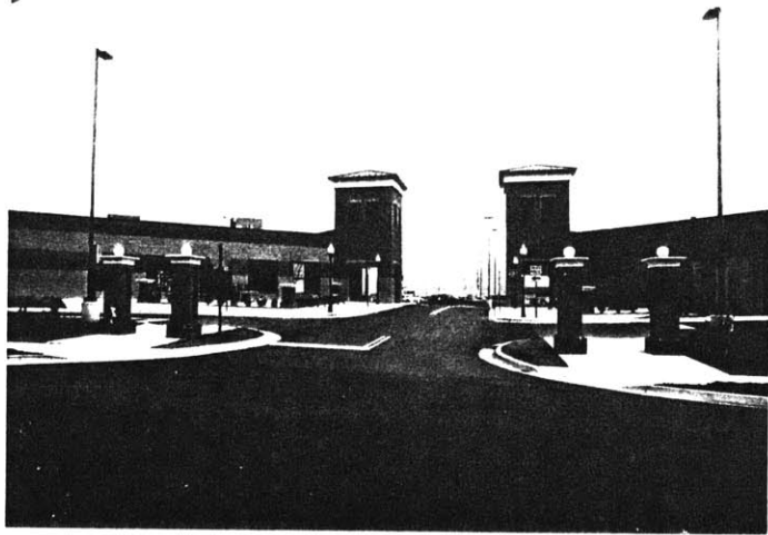
Figure 3-7: Existing mall at Kentlands. Pedestrian connection to residential district (12/25/94).
