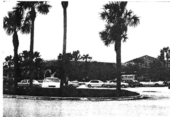
Figure 3-10: Shopping "plaza" in Florida. Includes lush landscaping and subdued sign graphics, but is still an isolated shopping center along a busy strip (1/4/95).
