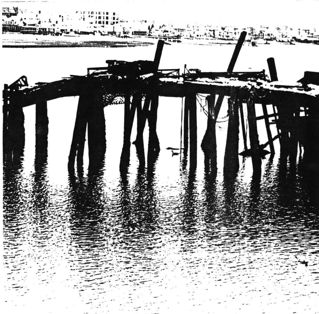
rotting piers P-town
