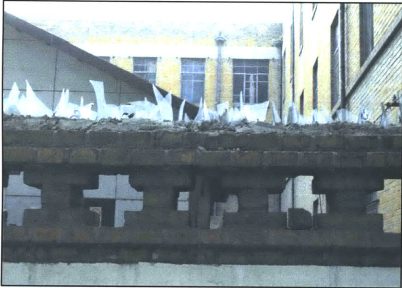
Detail of the wall
