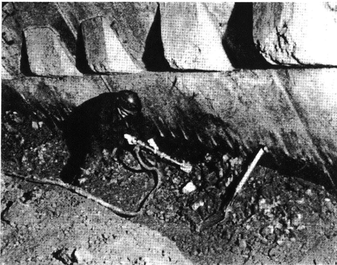
Figure 5-25 Manual excavation of soil within pneumatic chamber (from Megaw and Bartlett, 1982)
