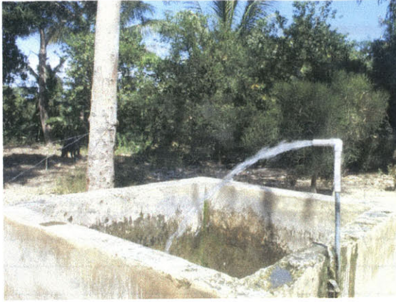
Figure 7 Examples of a free flowing captage (Dumay 5) and a fauceted captage (Bas Limbe 2).
