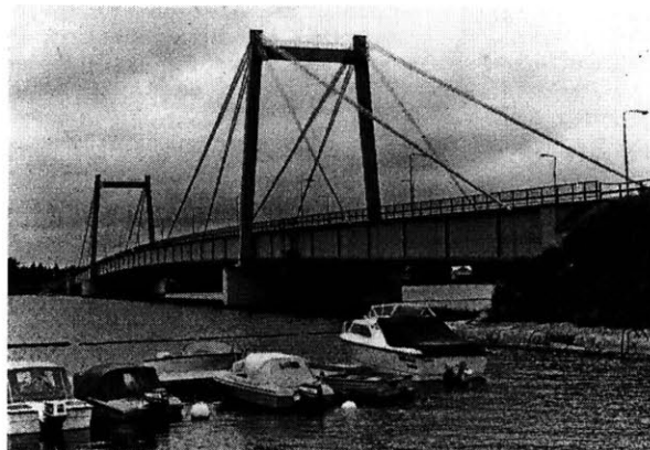
Figure 2.2 Strömsund Bridge [Gimsing, 1983]
