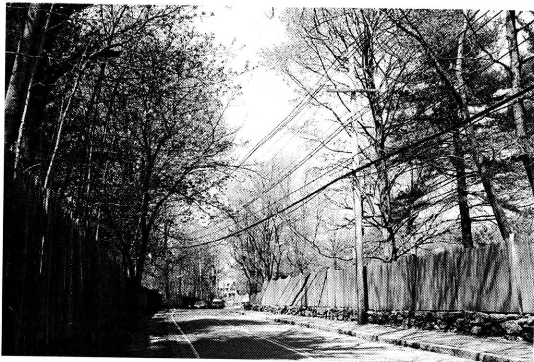
Near 185 Warren Street : The eruv switches with the utility lines from the left side to the right side.
