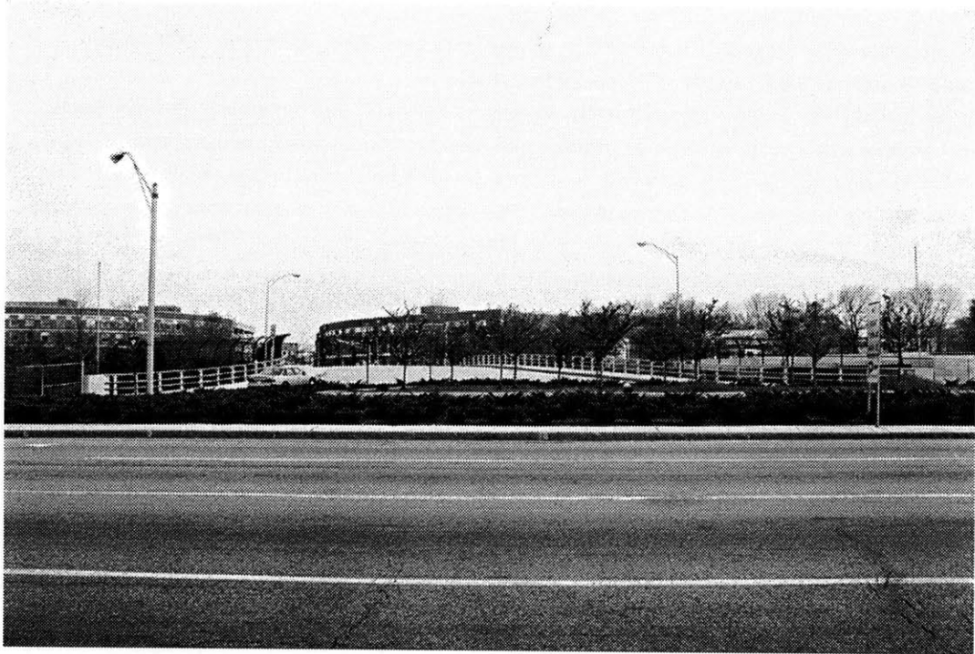
Intersection of Mass. Turnpike fence and overpass from Washington and Park Streets: As the two Street merge before they cross over the Mass. Turnpike there is a simple doorframe again with two poles on each side of the fence and a wire stretched between them. Both poles do not connect to the fence, so each pole has a small metal rod that connects the poles to the fence.
