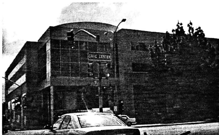
Fig. 28 Image of existing adjacent office
