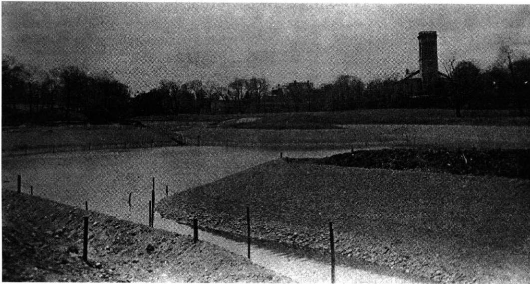
Figure 3.15 Muddy River under construction, 1892.
