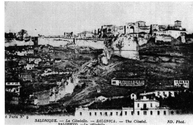
The upper part of the walls of Thessalonike and the fortress of the Acropolis in a photograph taken probably in the 1910s – compare with El Greco's Toledo in a tempest .
