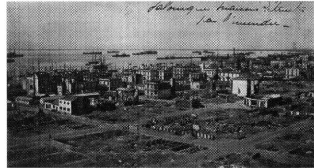
The south part of the city center photographed a few months after the fire. The rubble has been cleared up for the implementation of Hebrard’s plan.
