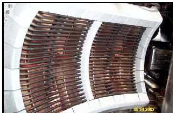
Figure 3-4: Picture of J-Antenna as installed in the vacuum vessel.
