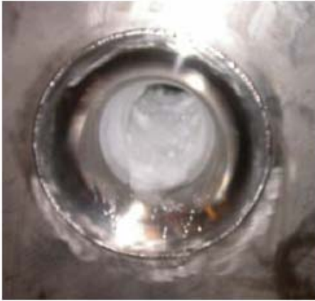
Condition of the Dished Head end Bore April 4 2006. There is a substantial ice build-up. This accumulated over the couple of weeks that the magnet was cold.
