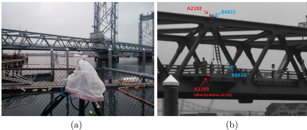
Figure 7-10: (a) Picture of the view from the camera for the December 14, 2015 measurement with (b) screenshot from the recorded video with comments as to the locations of the accelerometers and strain gauges on the bridge
