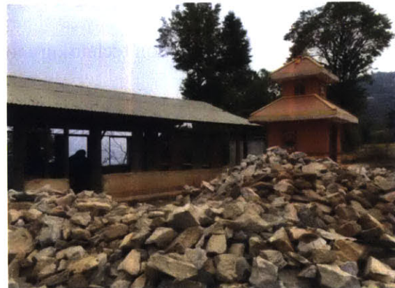
Figure 1-2: Collapse School Building in Kavre, Nepal
