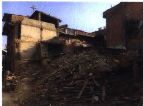
Figure 1-3: Collapse of Houses in Bugamati, Nepal
