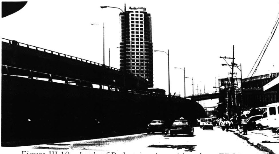
Figure III.10 Lack of Pedestrian Amenities along EDSA
