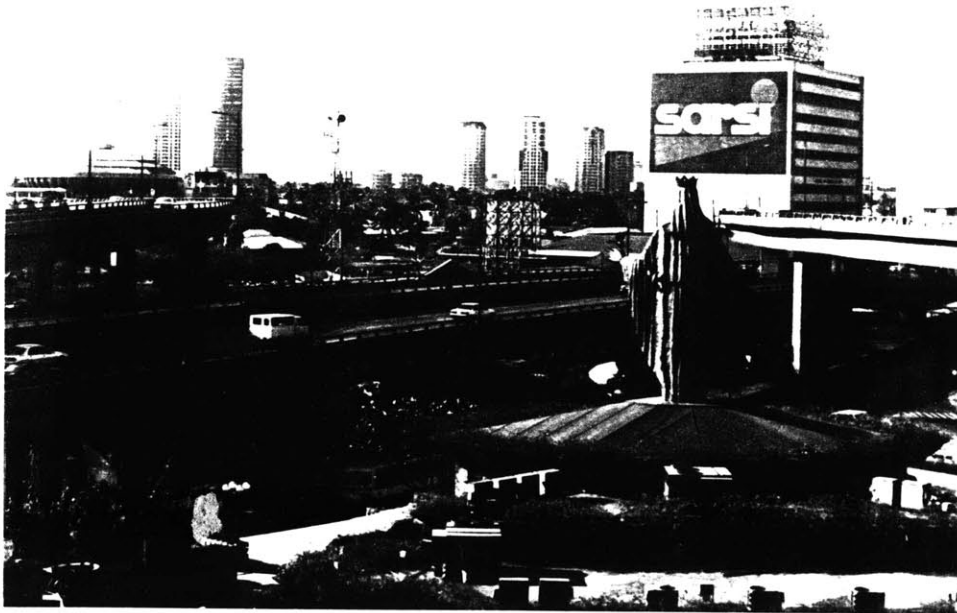
Figure III.5 Highway Overpasses along EDSA
