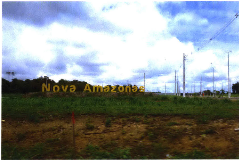
Clearing Land for New Housing Development
