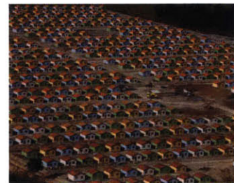
23 MCMV, Belo Monte Dam Construction Site, PA
