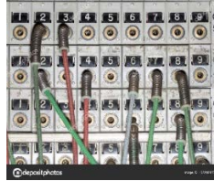
Fig 1: The old telephone switchboard may be conceptually analogous to future ‘plug-n-play’ integration platforms.
