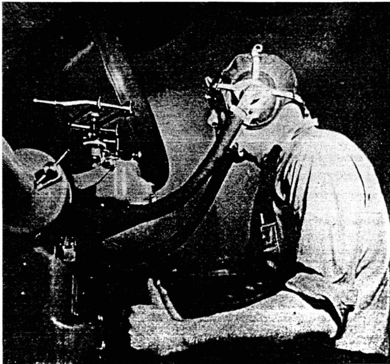
Figure 3-4a: Sperry Sound Ranging Equipment, human operator.
