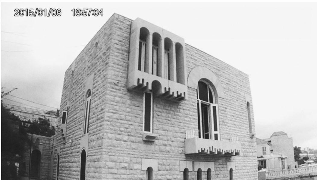
Figure 18 – Screenshot of a site survey video in front of the beach house in Halat, North Lebanon
