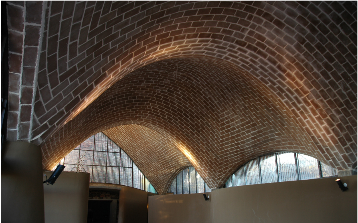
Fig. 1.7. Mapungubwe Interpretive Center, South Africa. Peter Rich Architects with John Ochsendorf, Michael Ramage, Henry Fagan, Philippe Block.
