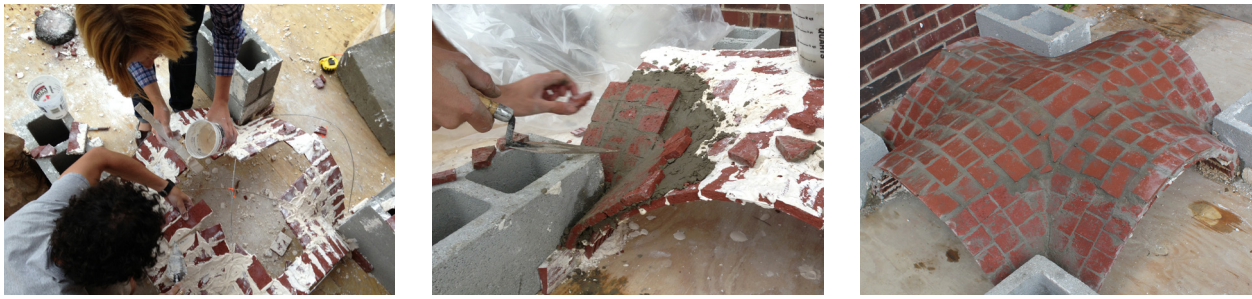
Fig. 0.4. Building a mini thin-tile groin vault in Philadelphia. From [Dessi-Olive, 2014].
