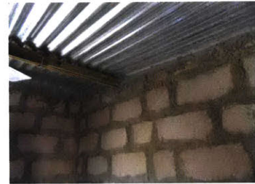
Tin Roof (R1)
