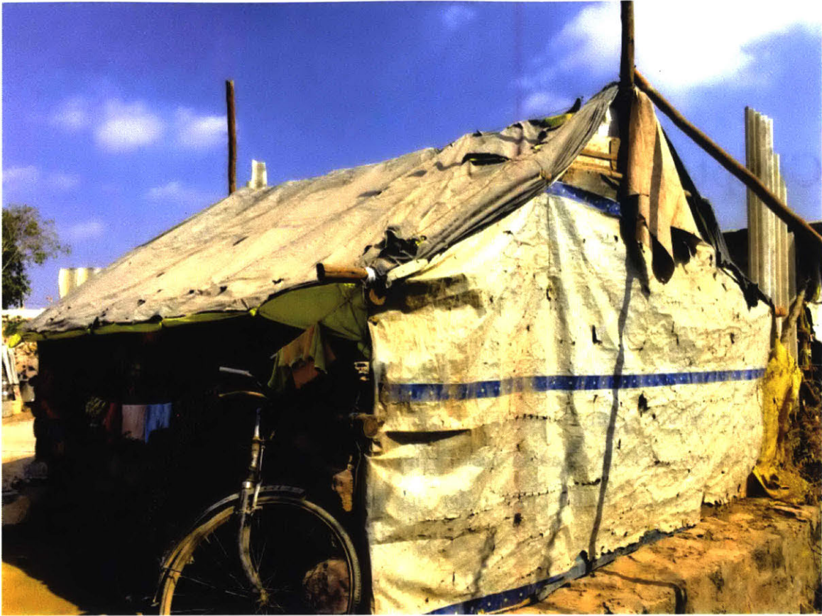
Figure 3-1: Exterior View of Informal Home (Photo Courtesy of Bradley Tran)
