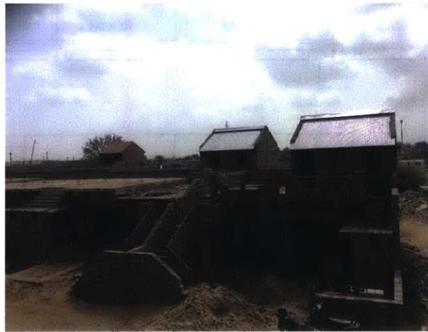
Housing for All Homes Construction
