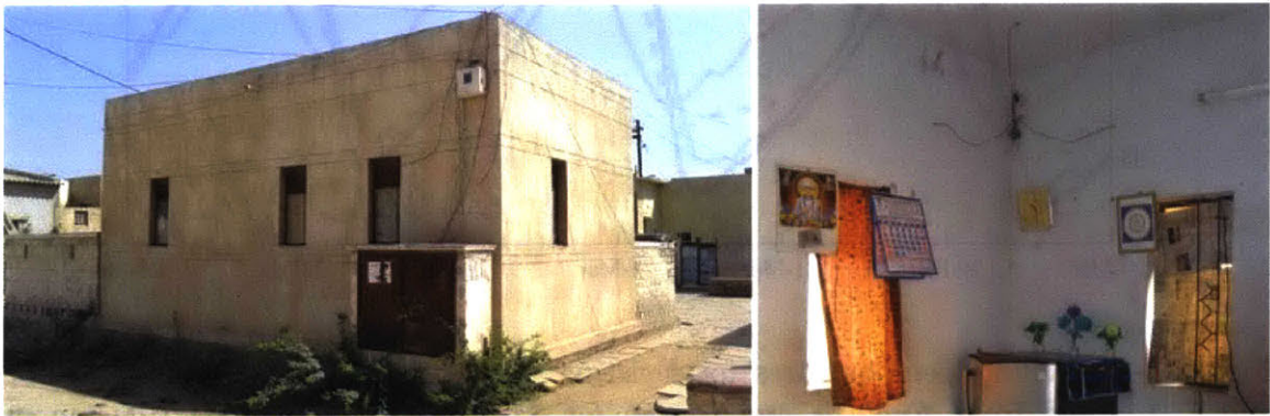
Figure 1-7: Single-Room Dwelling with 23cm Thick Uninsulated Compressed Stabilized Earth Block (CSEB) Walls and 12cm Thick RCC Slab Roof (Gradillas, 2015)
