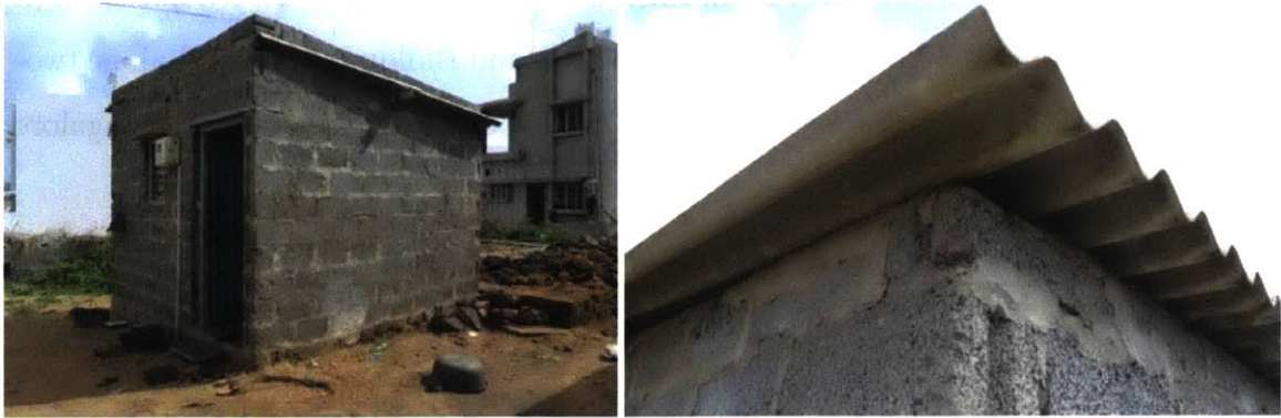
Figure 1-6: Single-Room Dwelling with 15cm Thick Solid Concrete Masonry Unit (CMU) Walls and a Bare Asbestos Cement Corrugated Sheet Roof (Gradillas, 2015)
