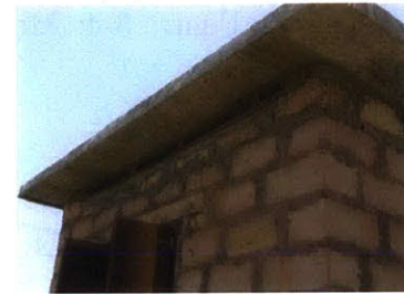
RCC Roof (R2)
