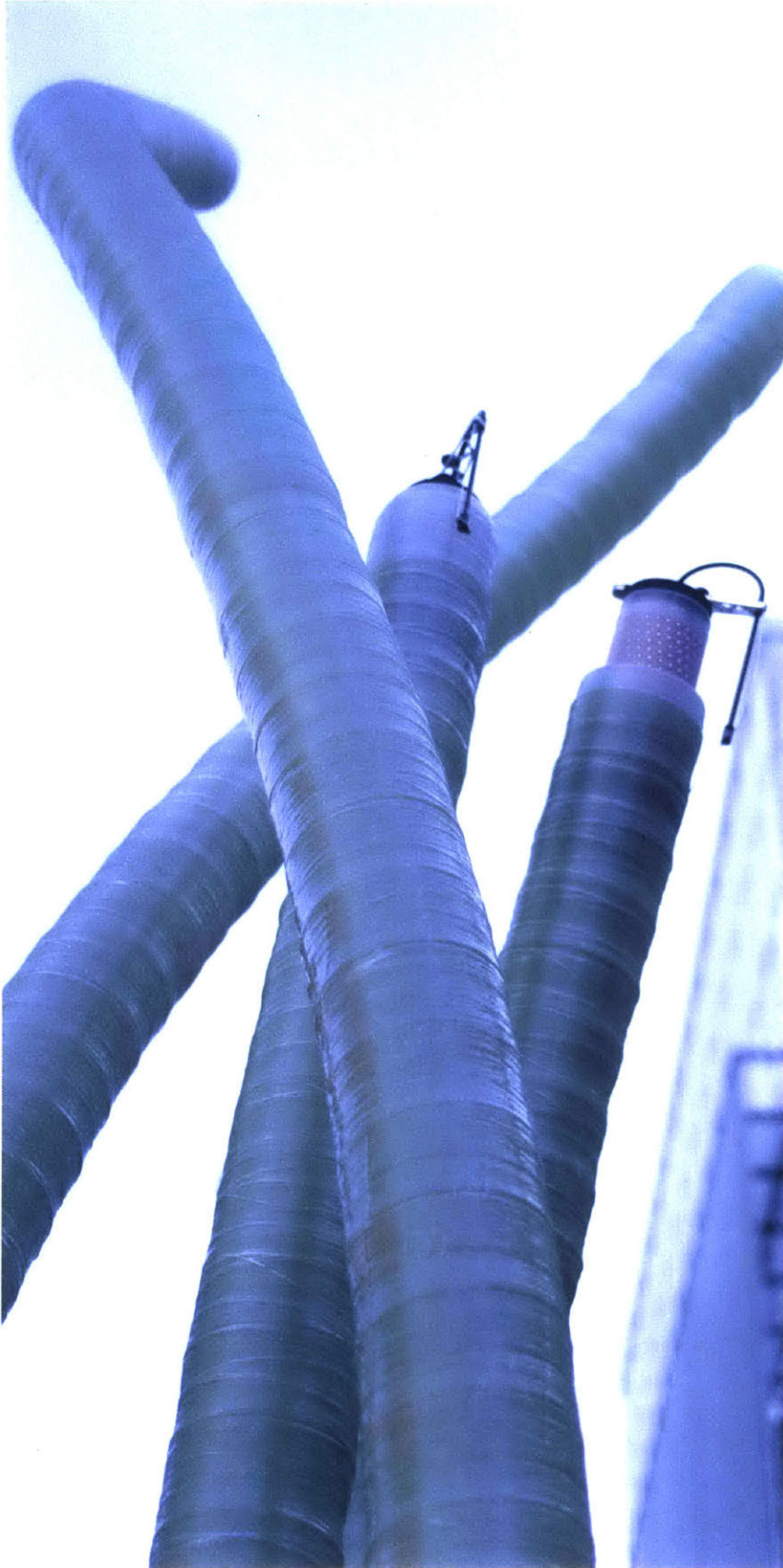
Figure 7.84: Columns being erected by the Fiberbots.
