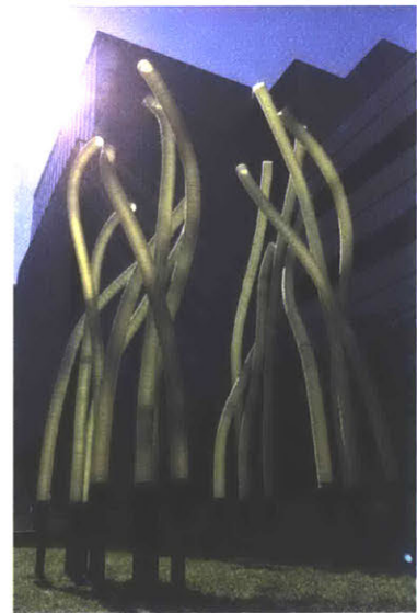
Figure 7.72: Finished structure in sunlight, showing translucency through the glass fiber tubes
