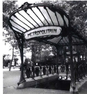
Figure 1.1: Entrance to the Abbesses Metro station (1900-4) by Hector Guimard, Montmatre, Paris Image by Steve Cadman, (Cadman 2007)
