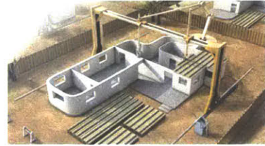
Figure 2.7: Illustration of the ‘Contour Crafting’ large-scale 3D printing method. Image source from: (Scott 2017)
