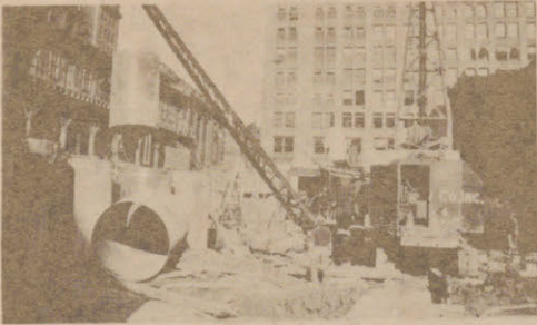
1. SWINGING CAISSON TO POSITION
