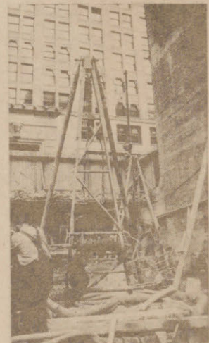
9. PULLING CAISSON AS CONCRETE IS CAST
