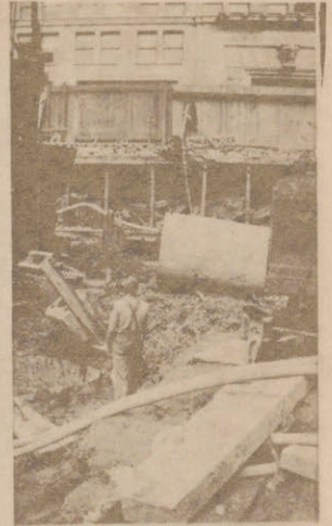
3. PICKING UP CAISSON HAMMER
