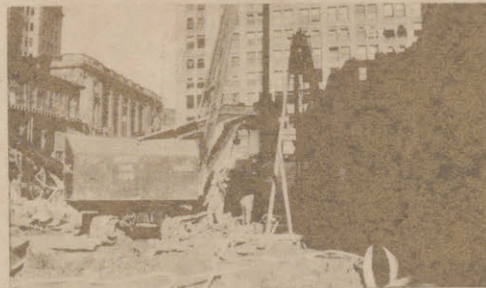
5. HAMMER DOWN ON CAISSON
