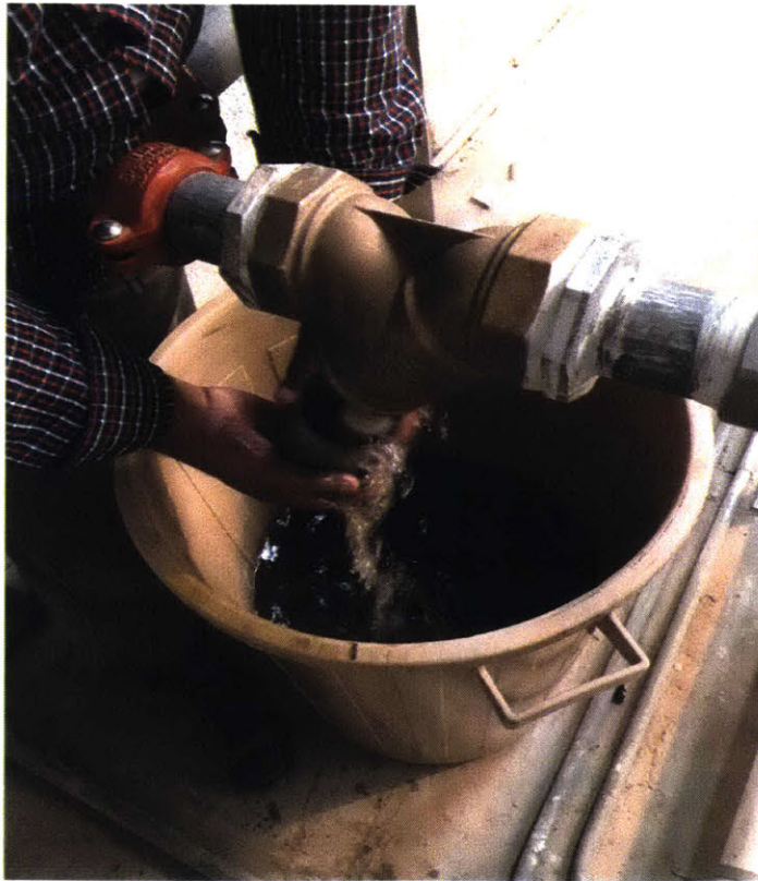
Figure 2-15: Example of the robot retrieval from a Y junction. The metallic mesh, in the shape of a tube, traps the robot inside. The mesh and the robot are being taken off the pipe system in this picture.
