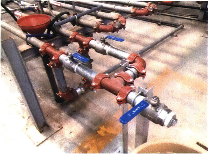
Figure 2-13: Example of the by-pass built for robot insertion.
