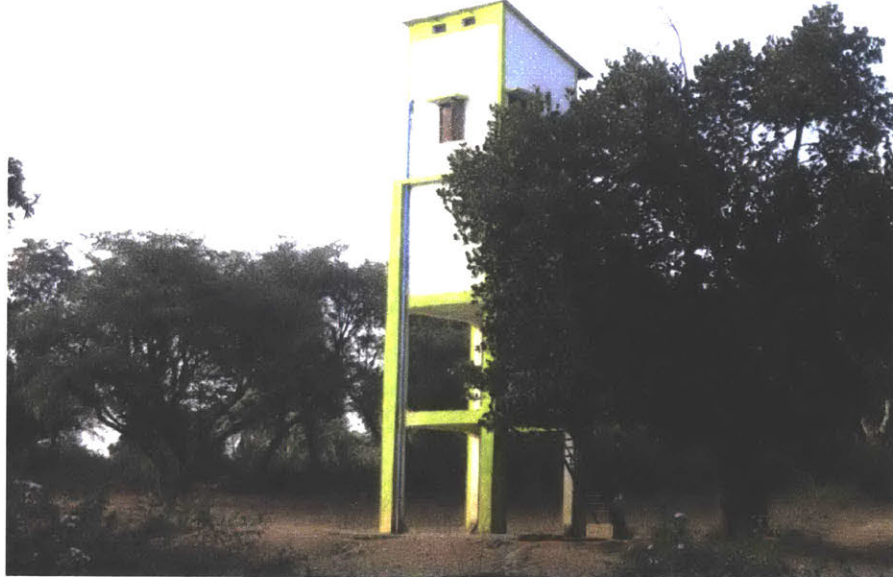
Water Tower in Ronhe, Jharkhand
