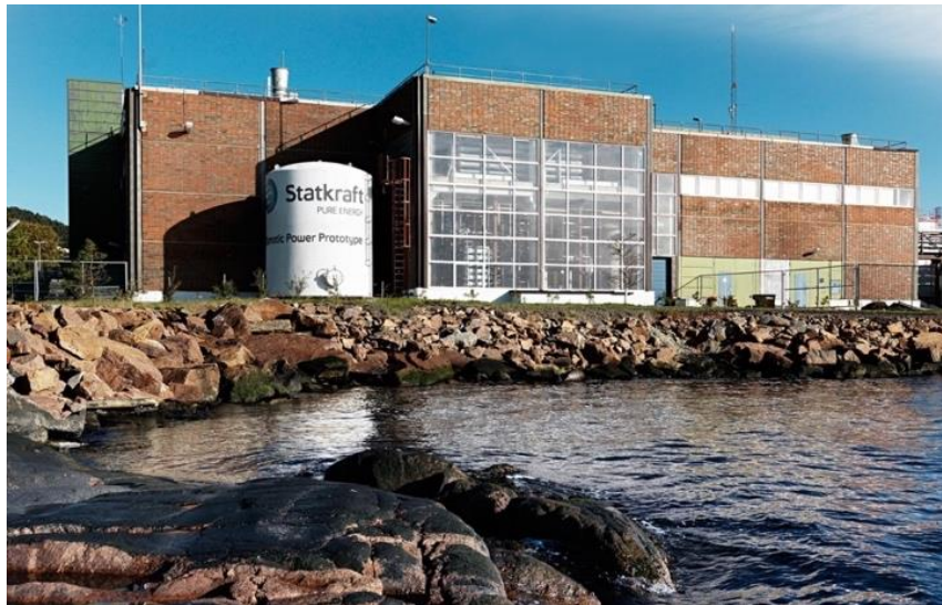
Figure 0-3: Statkraft PRO Power plant in Tofte, Norway [17]
