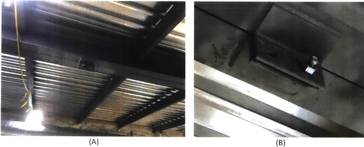
FIGURE 2.10- INTERMEDIATE MODULAR FASTENER. (A) CONNECTION LOCATION (B) INTERMEDIATE BOLTED CONNECTION (IMAGES TAKEN BY THE AUTHOR)
