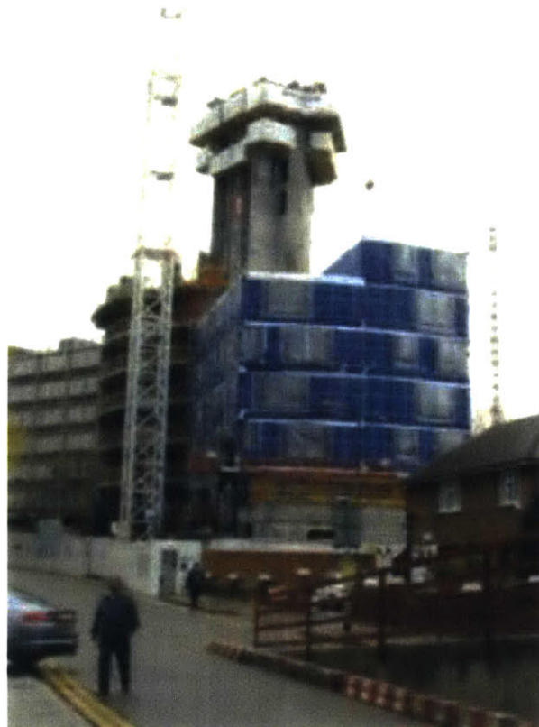
FIGURE 2.15- VICTORIA HALL CORE CONSTRUCTION (FUTUREFORM 2011)
