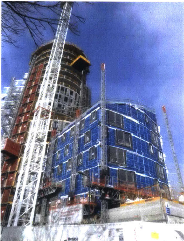
FIGURE 2.14 - VICTORIA HALL MODULE INSTALLATION (FUTUREFORM 2011)
