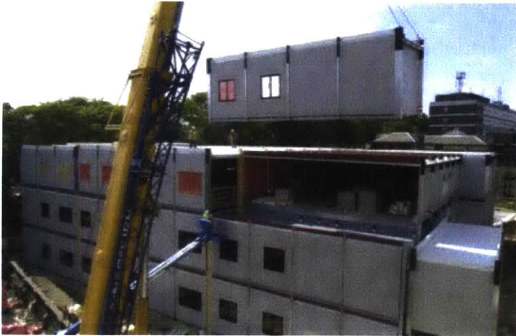
FIGURE 1.3 - INSTALLATION OF A MODULAR HOSPITAL (STEELCONSTRUCTION.INFO)
