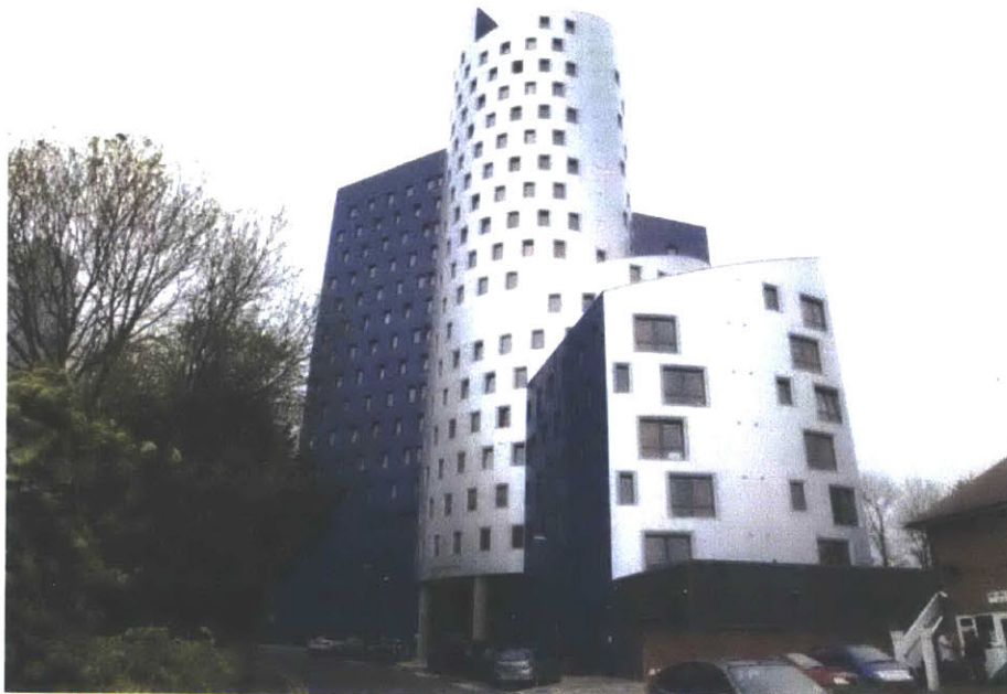
FIGURE 2.13 - VICTORIA HALL, UK (FUTURE FORM 2011)
