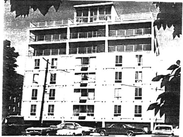
(Figures 2-1) Source; répertoire des systèmes de construction industrialisés en habitation. An example of "Kit of parts" (Componoform project). A structural system is divided into standardized precast concrete pieces.
