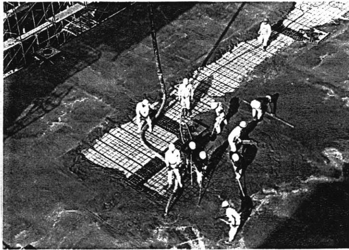
(Figure 6-16) Source: Toda Technics: Toda-Rahmen Precast Concrete Method Concrete casting
