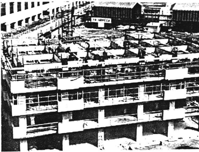
(Figure 6-12) Source: Kenchiku Gijyutu. Japan. December 1992. Construction of a high-rise multifamily buildup by the equal span grid system. (31 stories, 340 ft. Kagawa, Japan).
