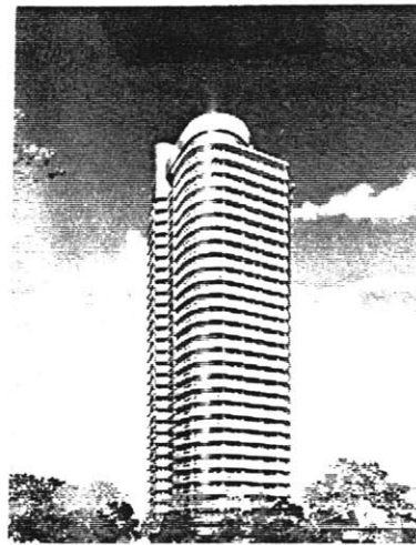
(Figure 6-12) Source: Kenchiku Gijyutu. Japan. December 1992. Construction of a high-rise multifamily buildup by the equal span grid system. (31 stories, 340 ft. Kagawa, Japan).
