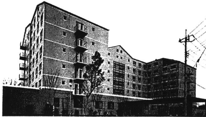
(Figures 4-1) Source: Toda Technics: Toda-Rahmen Precast Concrete Method The multifamily house constructed by the precast concrete braced frame structural system (7 stories, 99,000 ft 2 .) Beams, slabs, and external walls are precast, while columns are cast-in-place.
