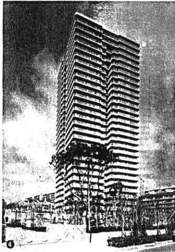
(Figure 6-7) Source: Monthly Building Engineering Magazine , January 1994, p.80. A multifamily house in Kawasaki, Japan. An example of a high-rise housing built by the equal span grid system (30 stories, 285 ft.). This project uses precast shell beam and slab. The strength of concrete is 420 \text{ kg/cm}^2 (5775 psi.).
