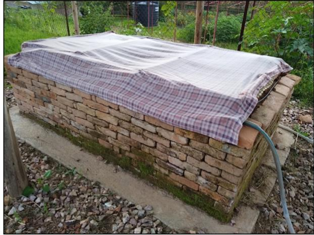
Above are images of a brick evaporative cooling device in Rubona, Rwanda.
