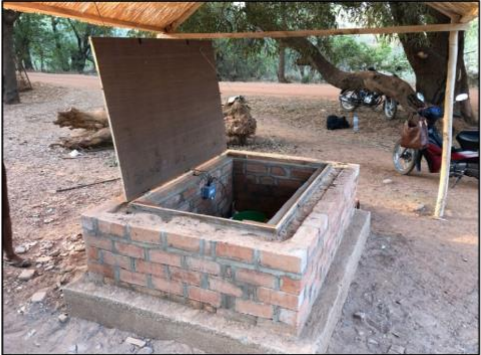
Above are images of a brick evaporative cooling device in Kamboinse, Burkina Faso.
