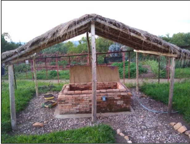
Above are images of a brick evaporative cooling device in Rubona, Rwanda.
