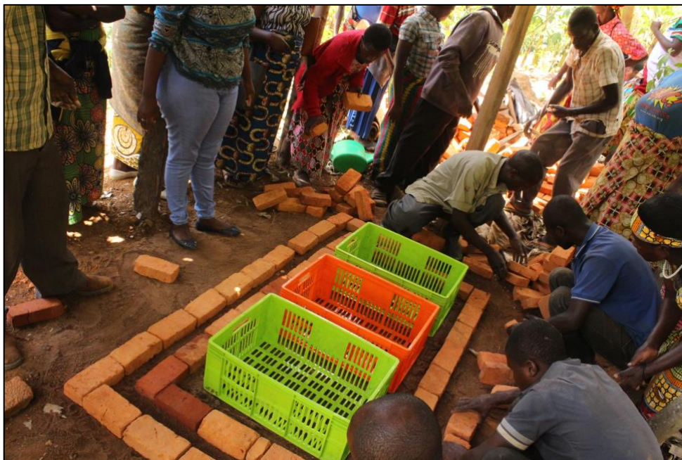
Figure 11. Construction of a brick Zero Energy Cooling Chamber by cooperative members in Gakenke, Rwanda.
