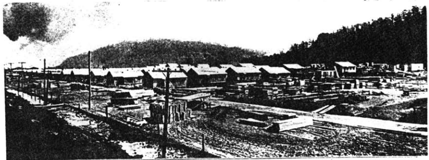
Sectional Houses Piled on the Ground Ready for Erection
