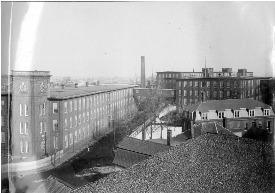
Figure 4.2: Naumkeag Steam Cotton Company buildings, December 1907. Source: Salem State University Archives, via Flickr: https://www.flickr.com/photos/salemstatearchives/46210293832
