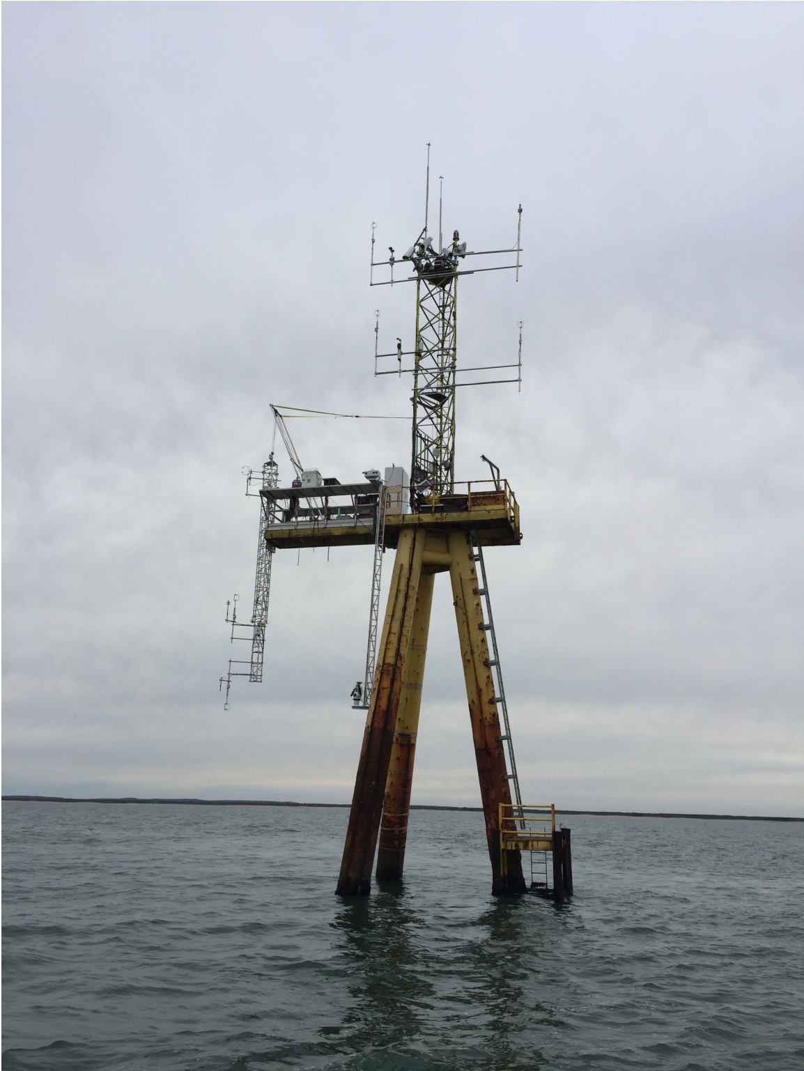
Figure B-1: ASIT met-tower. Windcube v2.0 (white box) is mounted on a platform 13 m above mean sea level.
