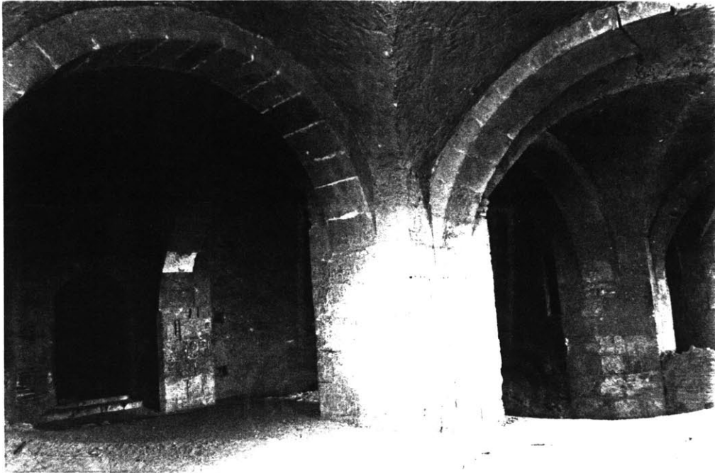
Fig 4. 11 View of One of the Barrel Vaults.
