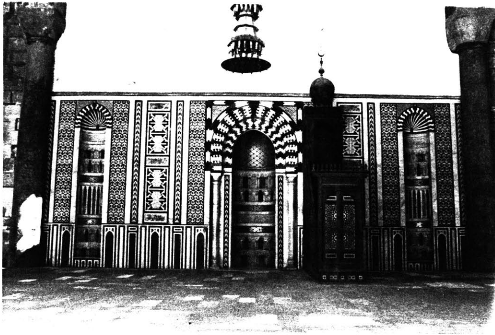
Fig 4. 23 Marble Dado of the Mosque's Qibla Wall.
