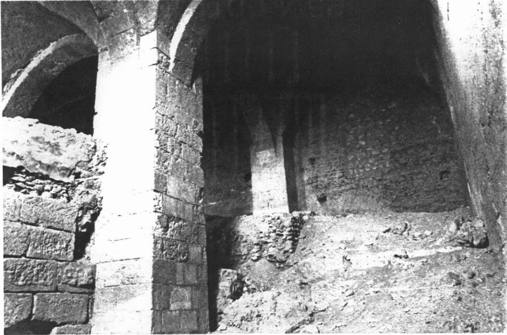
Fig 4. 13 View of the Slope.
