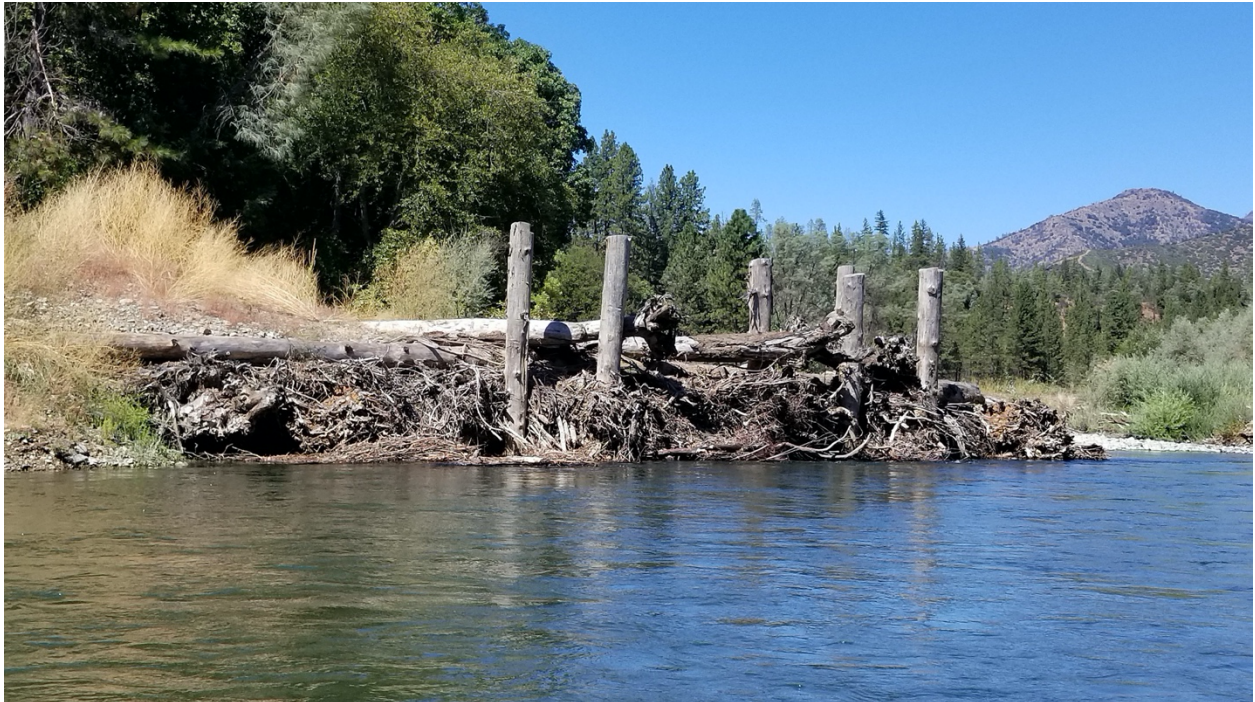
Figure 2: Engineered logjam placed in the Trinity River (Northern California). It was designed by the Yurok Tribe for restoration purposes (photo credit: D.J. Bandrowski). The vertical logs are the key logs to hold the logjam in place.
