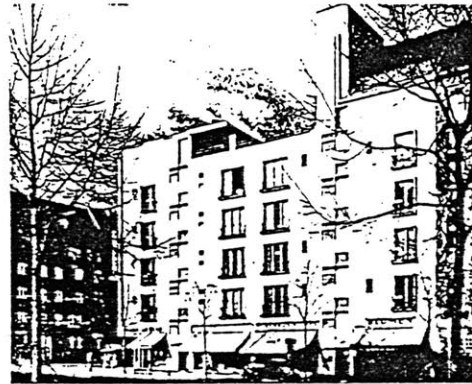
Figure 4-8: Kaiserdamm apartment block -1929.
