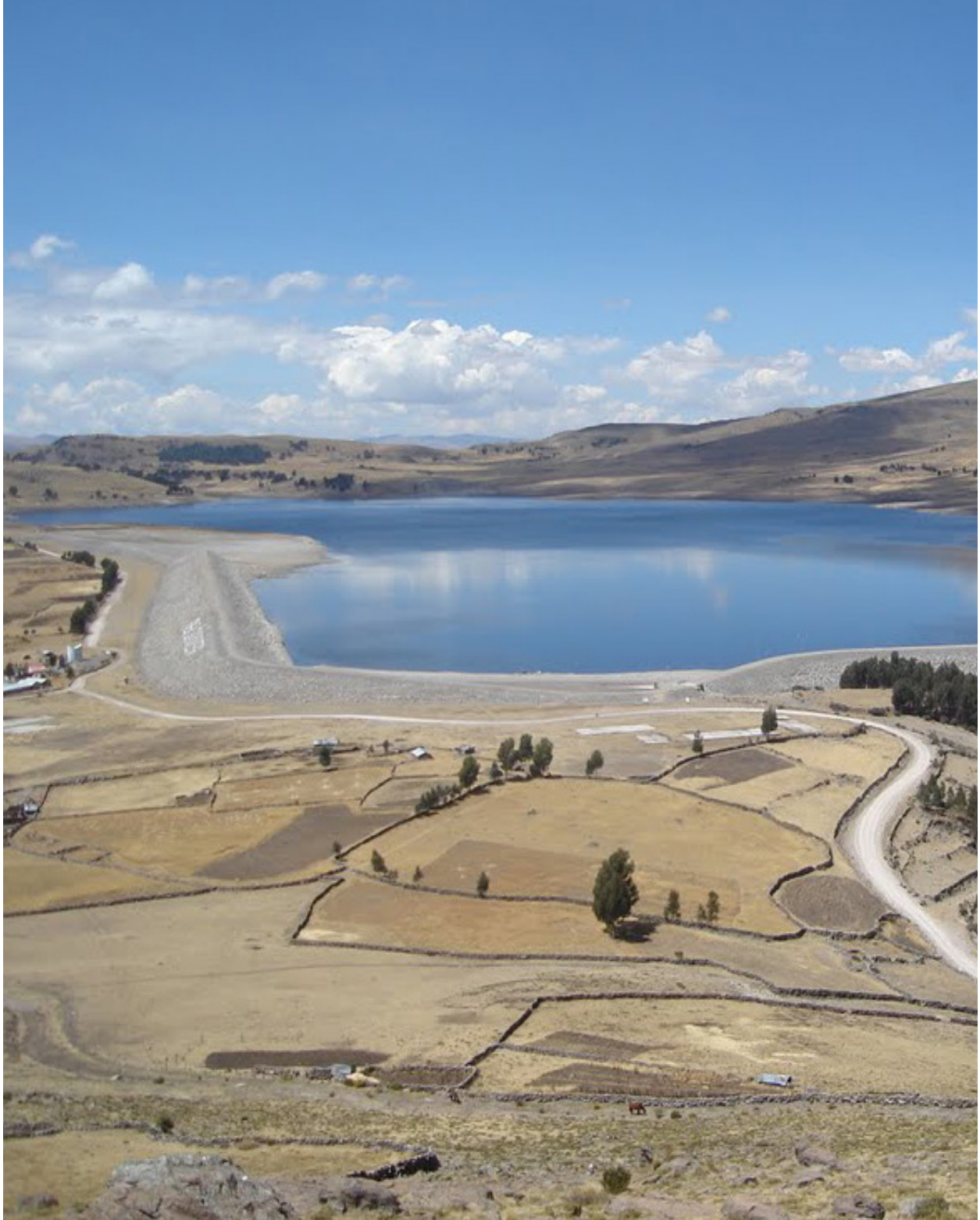
Figure 26 Cuchoquesera's Dam. Ruben de la Torre, "Presas Cuchoquesera 80 MMC Estructura Mayor de la Irrigacion Cachi Ayacucho Perú", Mapio, Accessed April 24, 2023, https://mapio.net/pic/p-36347730/
