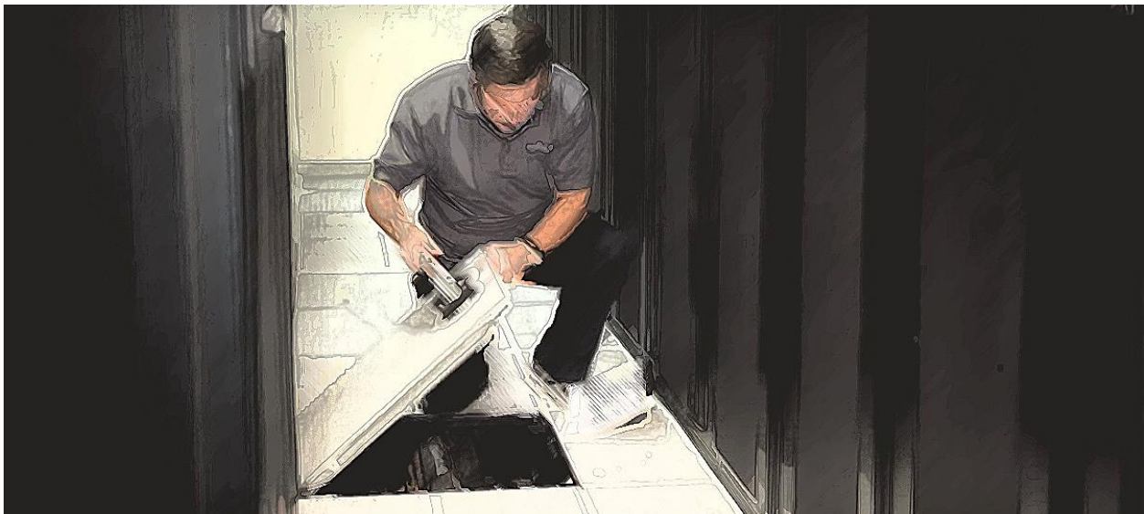
Tom Haines pries open floor tiles to increase airflow from underfloor, Image: Artistic Render by Author
