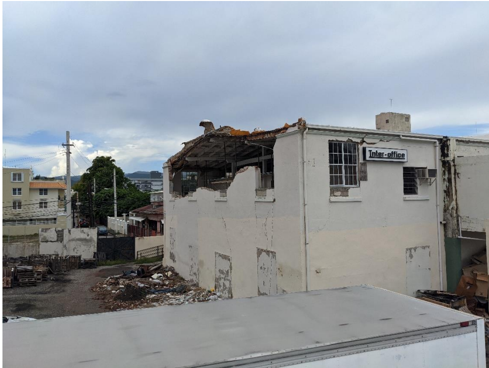
Earthquake damage to buildings near Ponce Data Center, Image: Author
