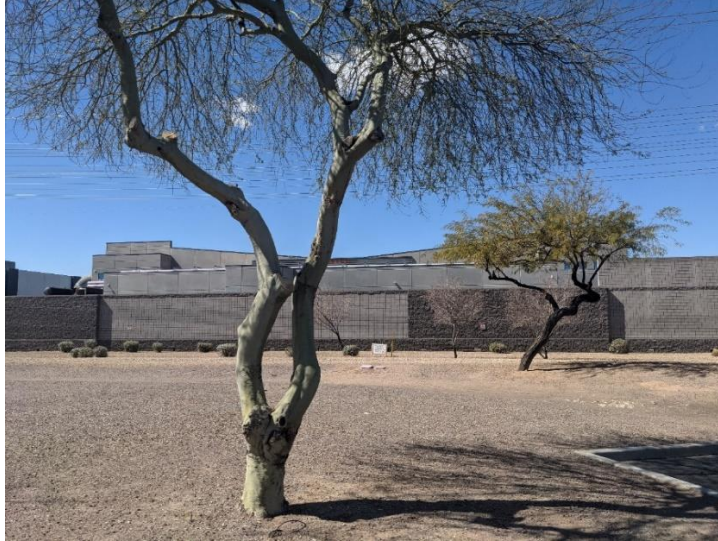
Cyrus One Data Center in Chandler Arizona, Photo by Author
