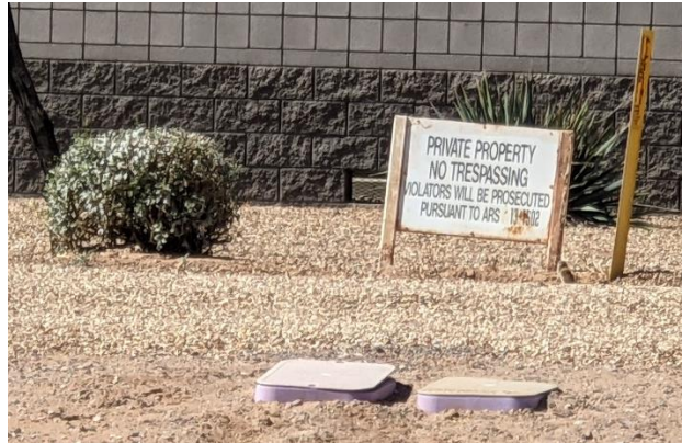
Cyrus One Data Center in Chandler Arizona, Photo by Author
