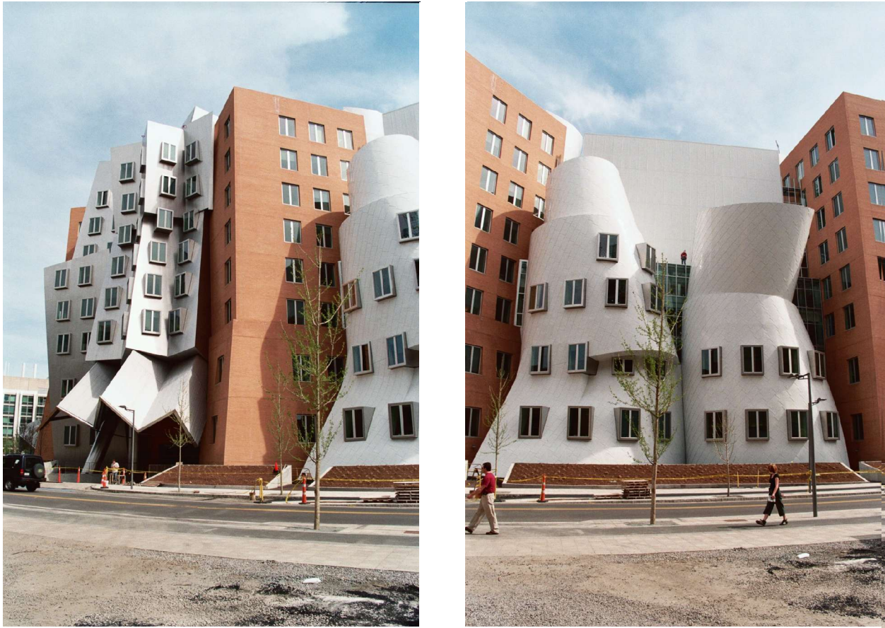
Figure 3.7 Two views of the Stata Center from Vassar Street.
