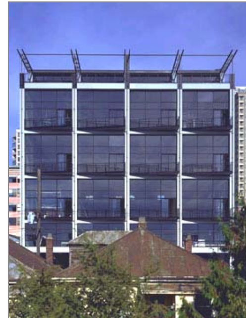
Figure 14: The Banner Building, Western Avenue frontage. (Weinstein Copeland Architects)
