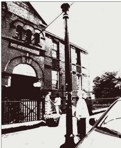
Figure 35: The Joshua Bates School, Harrison Avenue frontage. (date and origin unknown)
