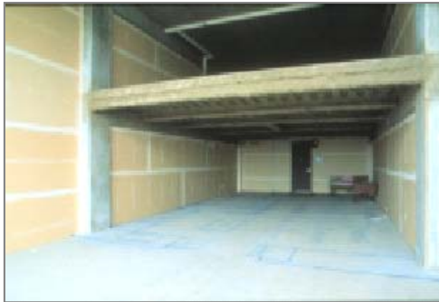
Figure 19: Unfinished live/work unit. (Koryn Rolstad)
