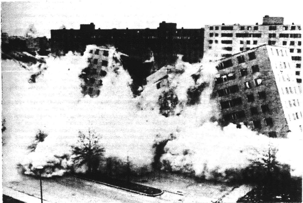
Figure 15: Demolition of Pruitt Igoe, St. Louis, 1971 ( Collage City, Rowe and Koetter, 1978 )
