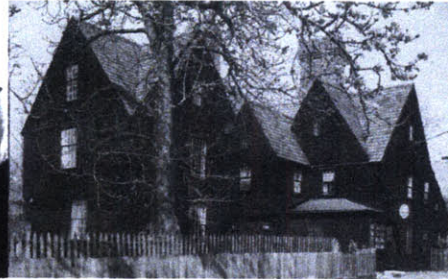
1700 - Colonists build as they would in their homelands, forming a collection of nomadic styles - Homes arose out of cultural and religious practices, geographic location, and availability of local materials
