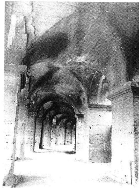
Figure XXXIV: Concrete vaults in the Colosseum ambulatories
