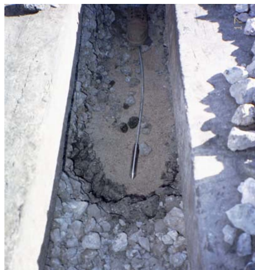
Figure 5.17: Installing settlement probe 2 from the top of ballast
