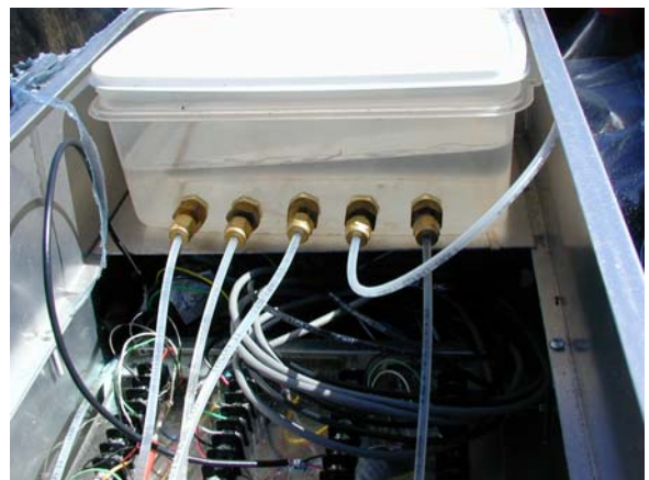
Figure 5.25: Reservoir for the settlement probe
