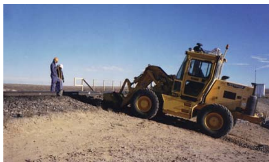
Figure 5.18: Excavation of the rail ballast using a front-end-loader
