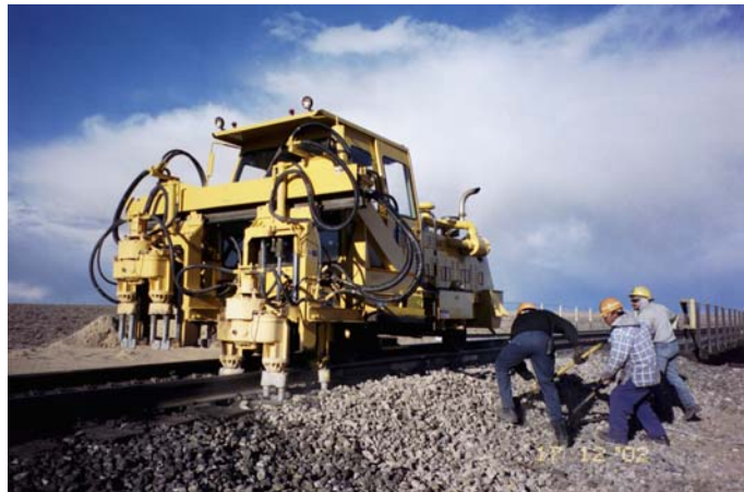
Figure 5.21: Compaction process of the ballast after installation of the probe.
