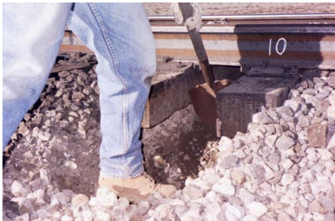
Figure 5.16: Excavating the top of the ballast by shovel.
