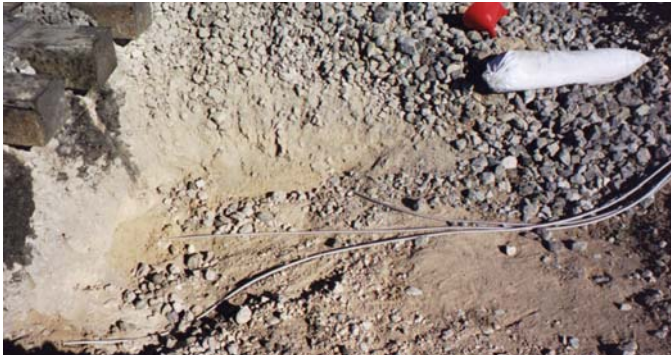
Figure 5.19: The augered hole is back-filled with sand.
